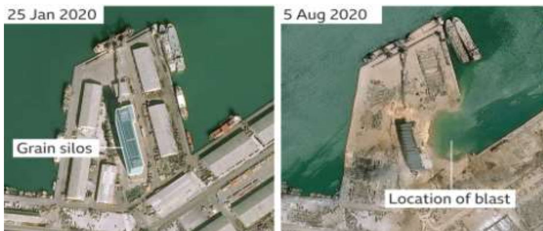
FIGURE 1: BEFORE-AND-AFTER IMAGES OF THE PORT OF BEIRUT.
